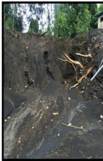
FIGURE 1B. LANDSLIDE LOCATIONS IN PENELOKAN VILLAGE, SUB DISTRICT OF KINTAMANI
