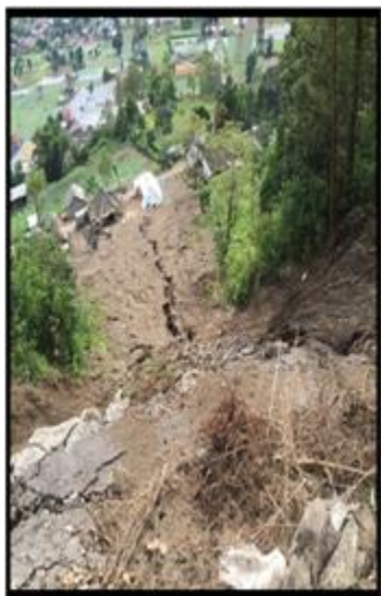
FIGURE 1A. LANDSLIDE LOCATION IN SONGAN VILLAGE, SUB DISTRICT OF KINTAMANI
