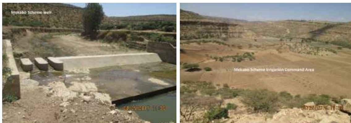
FIGURE 1. The weir and irrigation command area for Mekabo small- scale irrigation scheme
