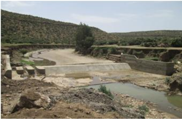
FIGURE 2. CONSTRUCTED WEIR TO DIVERT WATER TO MEKABO SMALL-SCALE IRRIGATION SCHEME
