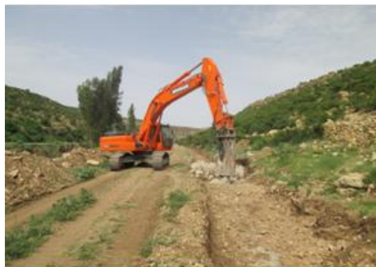
FIGURE 4. MEKABO CONVEYANCE CANAL PRESENTLY UNDER CONSTRUCTION
