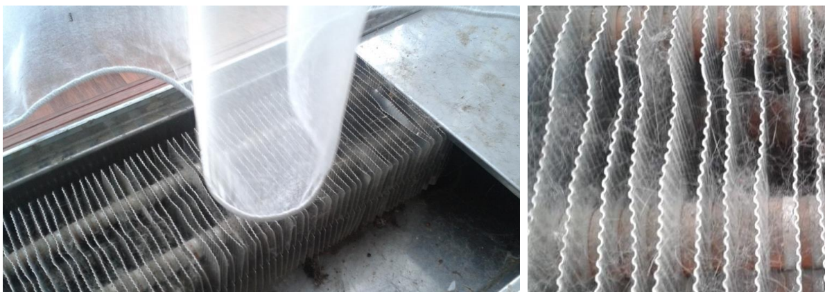
FIG. 5: FLOOR LAMELLAE CONVERTOR OF ROOM OF A FLAT WITH A CAT (TWICE A YEAR CLEARED); DISTANCE OF THE CONVERTOR LAMELLAS IS 3 mm
