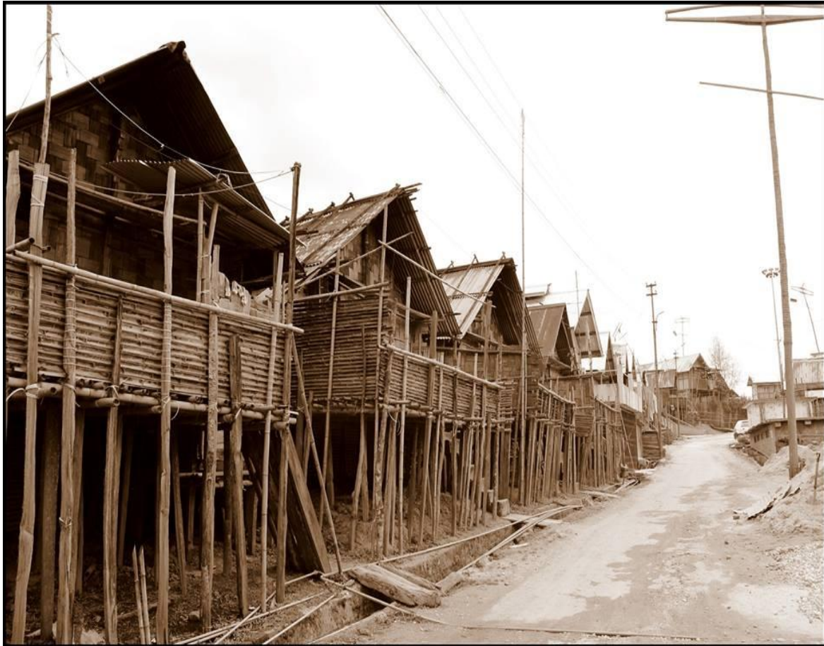
FIGURE 3. NEWLY CONSTRUCTED TRADITIONAL HOUSES OF THE APATANI TRIBE IN ZIRO VALLEY OF ARUNACHAL PRADESH, INDIA. THE SUPPORTING STRUCTURES OF THE TRADITIONAL HOUSES ARE MADE UP OF PINE TIMBER WHILE FLOOR, WALLS AND ROOF ARE CONSTRUCTED OF P. bambusoides
