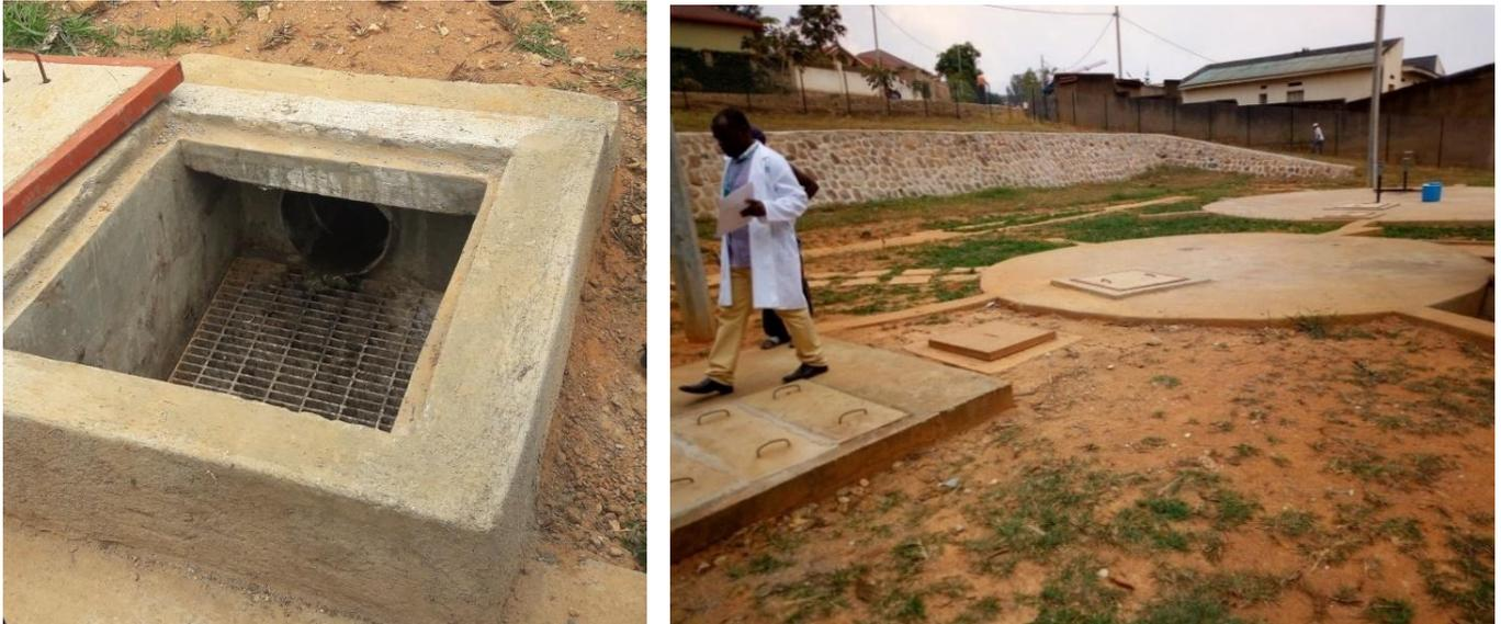
**FIGURE 1: Pre-treatment unit (a), Primary settler, Bioreactor, secondary settler (b)**
