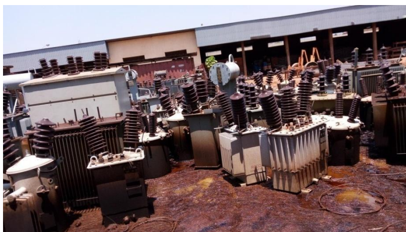
FIGURE 2: Contaminated site of Gikondo/Industrial Park
